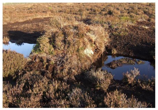
**Plate 5.** Example of use of a 'peat plug' in drain blocking – the plugs are placed at intervals along the drain and are highly effective in stemming water loss from the bog.
